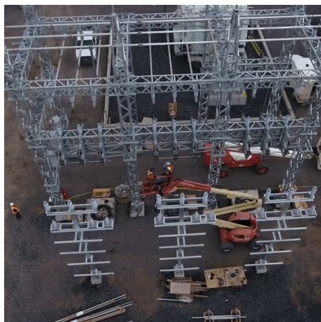
Construction of Clear River Energy Center | Invenery
